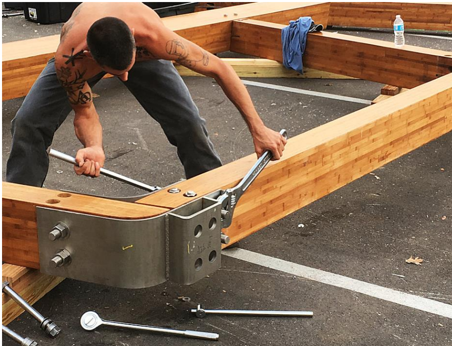
Engineered glulam beam made of Structural Engineered Bamboo (SEB) incorporating stainless steel plating and hardware - Image Provided by ReNuTeg, Inc.
